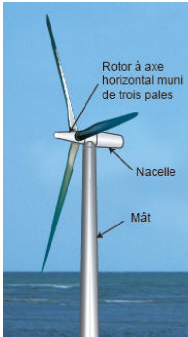
The components of a wind turbine
