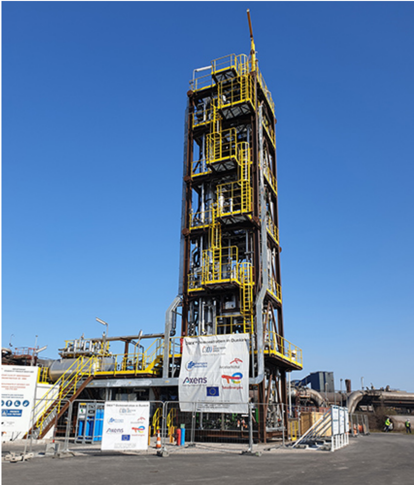
Image 1: DMX(TM) demonstrator on site of ArcelorMittal in Dunkirk. Acknowledgements: IFPEN
