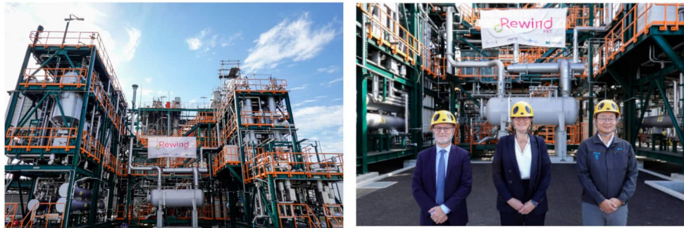
(Left) Exterior view
